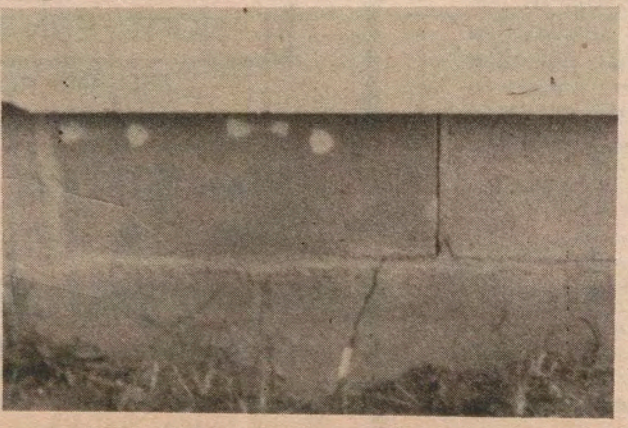
Foundation cracked
