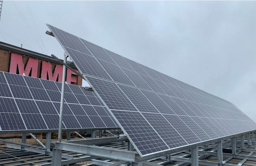
Photovoltaic panels have been installed on the roof to convert solar energy into usable electrical energy.
